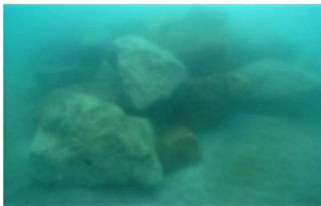
Seaweed bed created by installing natural stones
