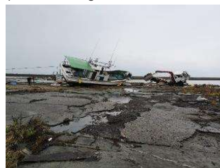
Pier damaged by the earthquake and a fishing vessel stranded by the tsunami (Ukai Fishing Port, Ishikawa Prefecture)
