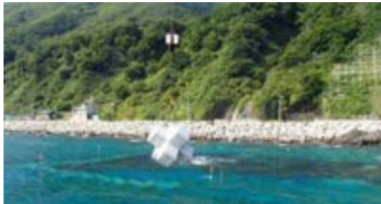
Seaweed bed creation (installation condition of blocks on which marine algae can easily take root)
