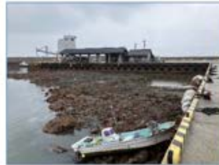
Damage to fishing ports (sea-bed uplift) and fishing vessel capsizing
