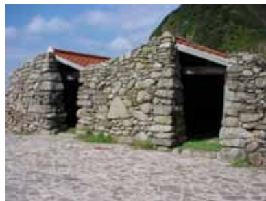
Funaya (boat storage), also referred to as mogoya (alga storage) built at a rocky beach without a wharf with piled beach stones and thatched roofs (Tsushima City, Nagasaki Prefecture).
