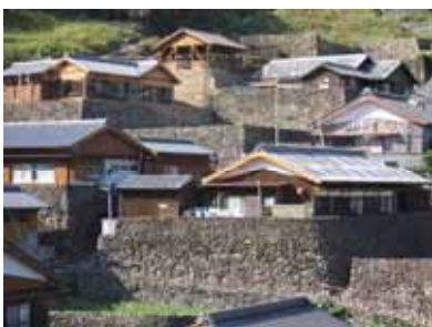
Stone walls built in the late 19th century to protect the houses in the fishing village from the strong northwestern wind in winter (Ainan Town, Ehime Prefecture).
