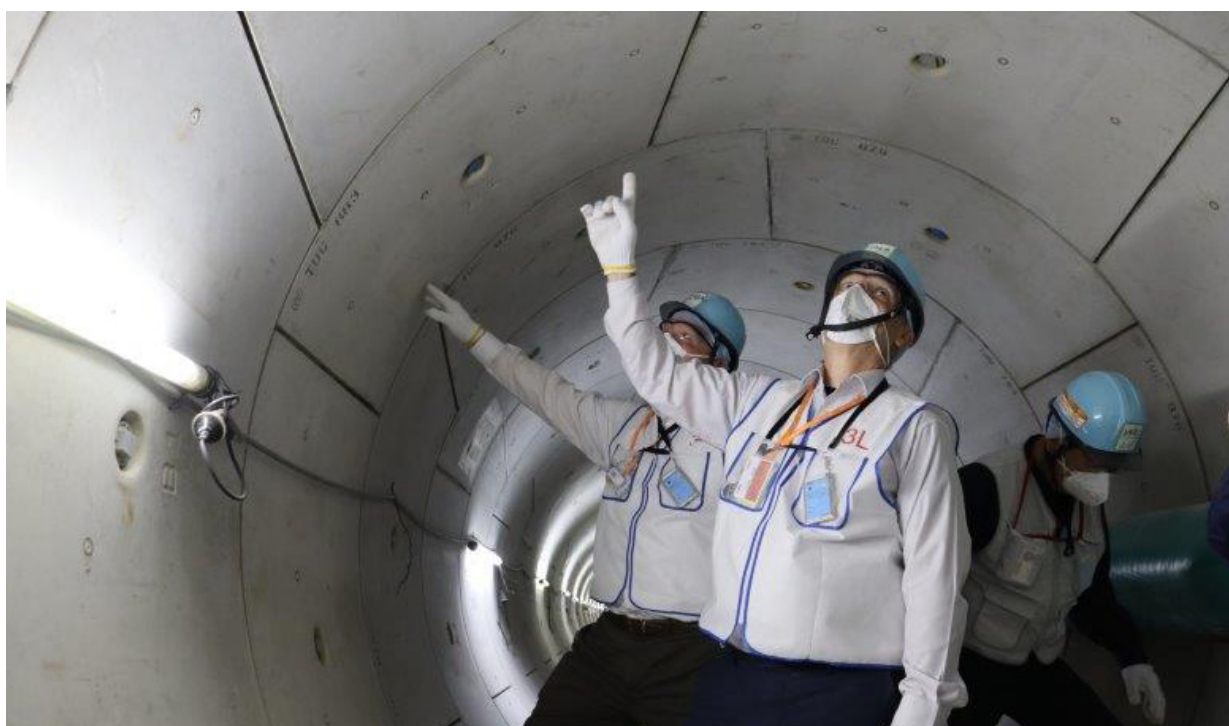
Figure 3.8. Pre-service inspection of ALPS discharge facility
